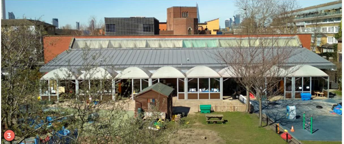
Anne Burnadt Nursery viewed from the application site
